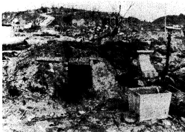
Fig. 1.5. Undamaged earth-covered family shelter in Nagasaki.
