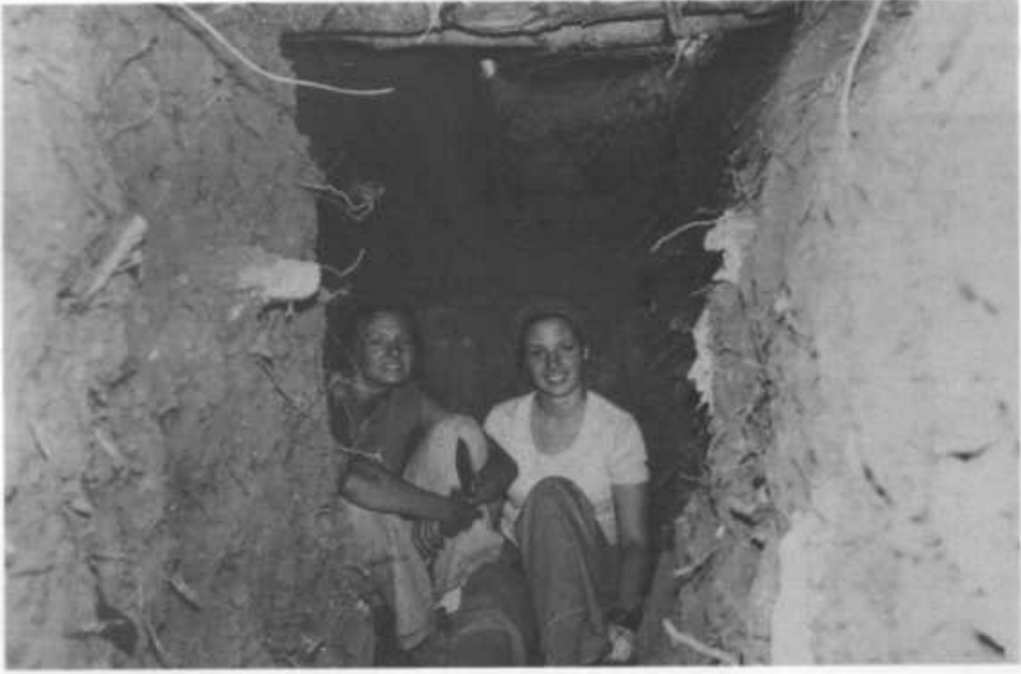
Fig. 5.2. Two non-athletic college girls who completed a 4-person Pole-Covered Trench Shelter in 35-1/2 hours, despite tree roots.
