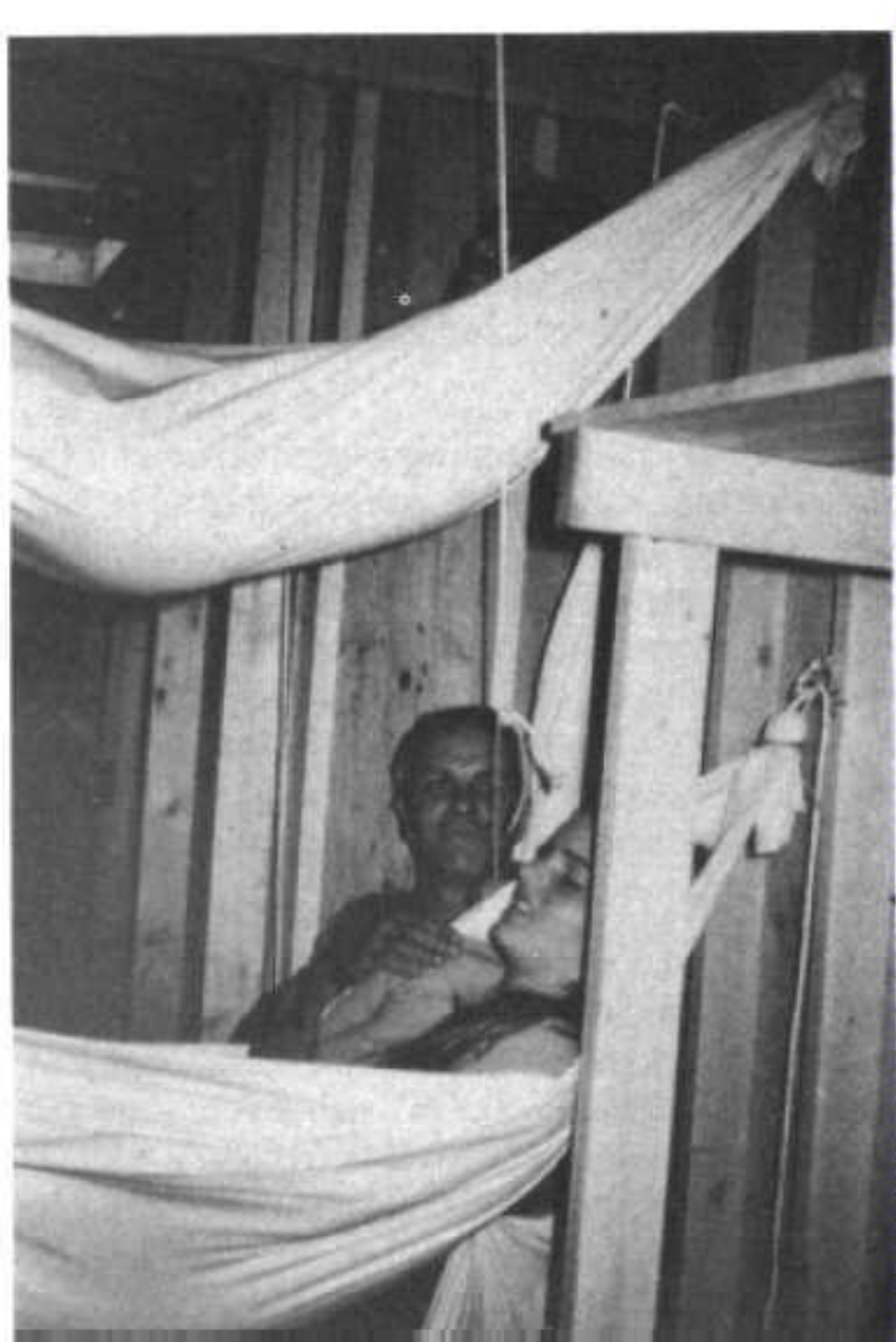
Fig. 14.4. Bedsheet-Hammocks hung one above the other across the room of a Russian-type Small- Pole Shelter made of lumber.
