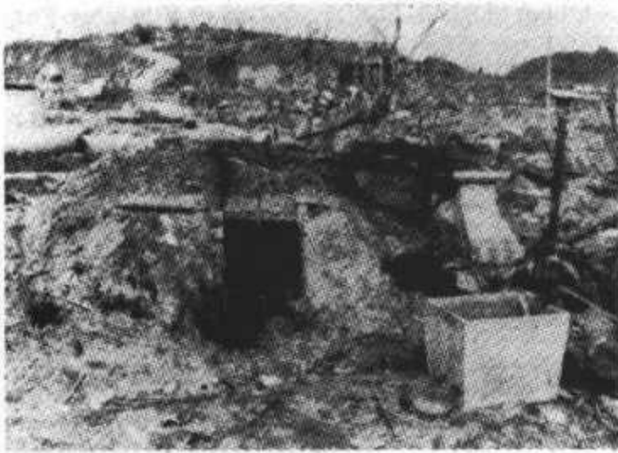
Fig. 1.5. Undamaged earth-covered family shelter in Nagasaki.
